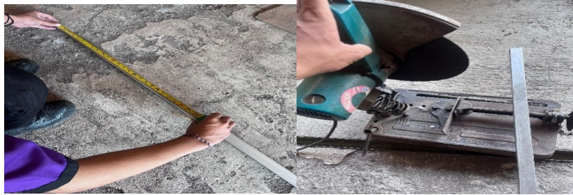
Figure 3. Steel Measurement and Cutting Process for Simulator Frame Construction
